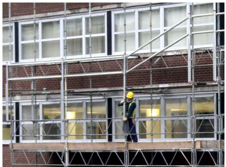
Turner Access Plus Guard System in use during scaffold erection
