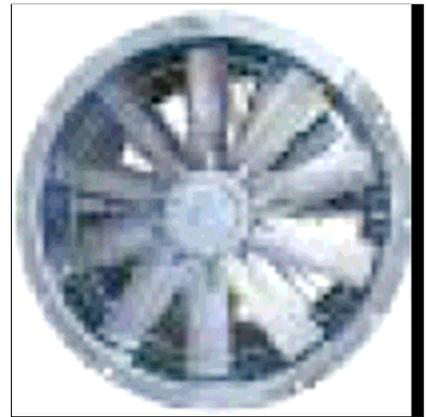
In systems such as a paint spray booth, an axial fan (see right) would be used, where the volumes are high but the pressure is low. Both are just as noisy!
