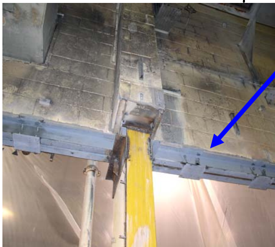
The finished job
